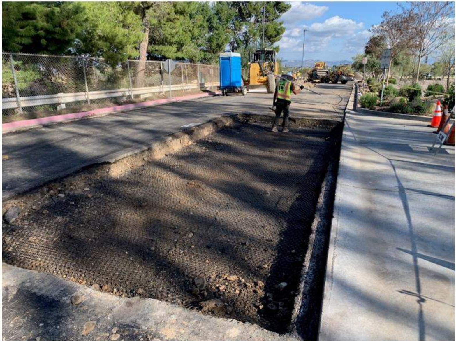
Phase 4 – Repair Area near Parking Lot 5 North Entrance
